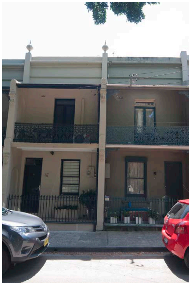
Detail, two of the Lackey Street terraces
