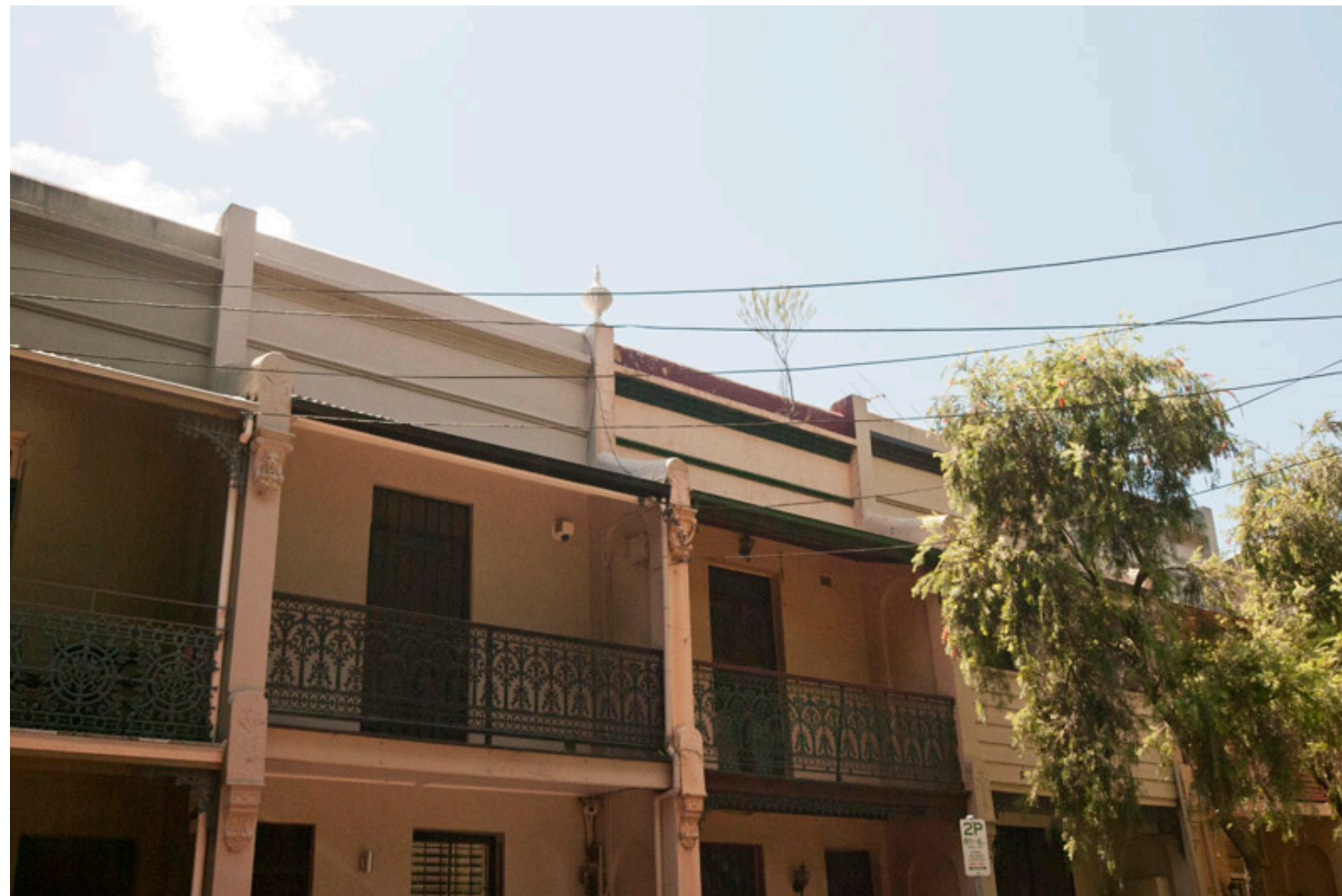
The parapet line of the Lackey Street terraces (note some urns missing)
